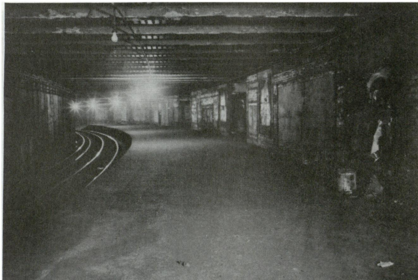
Photograph 9 Disused Wood Lane Underground Station (W London) lit partially by existing tungsten light and, in the foreground, by electronic flash
